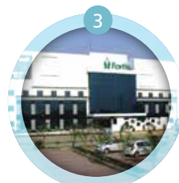
Fortis Hospital, Chandigarh Road, Ludhiana
